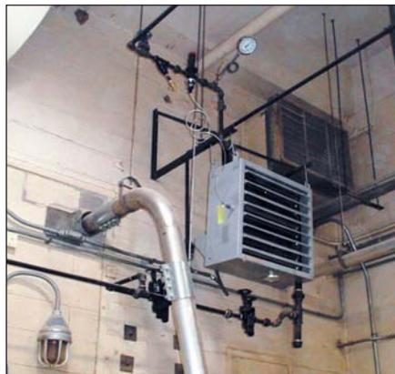
A permanently mounted steam heater in the sifting area of a Chicago, IL flour mill. Photo courtesy of Armstrong Intl. Inc.
